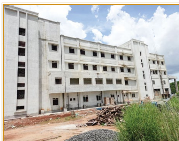
Burns Unit under Construction
